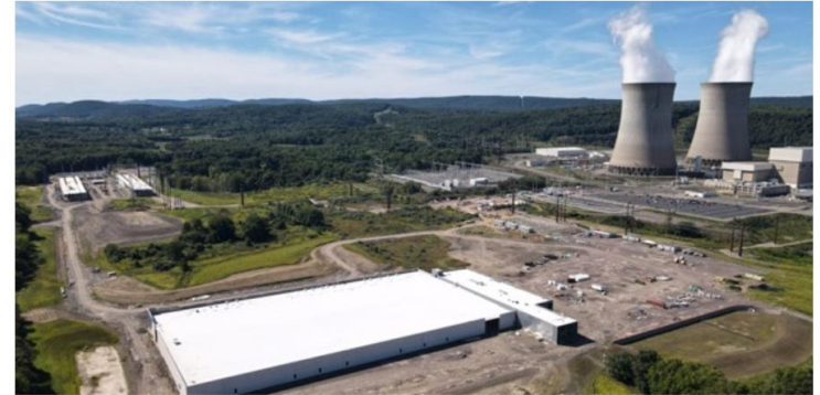
Susquehanna nuclear plant in Salem Township, Penn., along with the data center in foreground. (Photo: Talen Energy)
